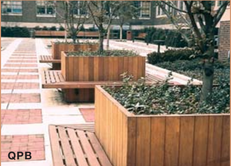
Standard widths: 18"; circular/square planter benches overall d or l 7'-11' Rect. planter benches: overall 48" l min. and 48" w -single, 66" w -double.
